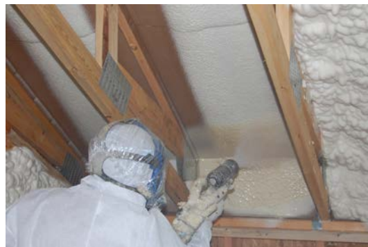
SPF being installed in an attic space
